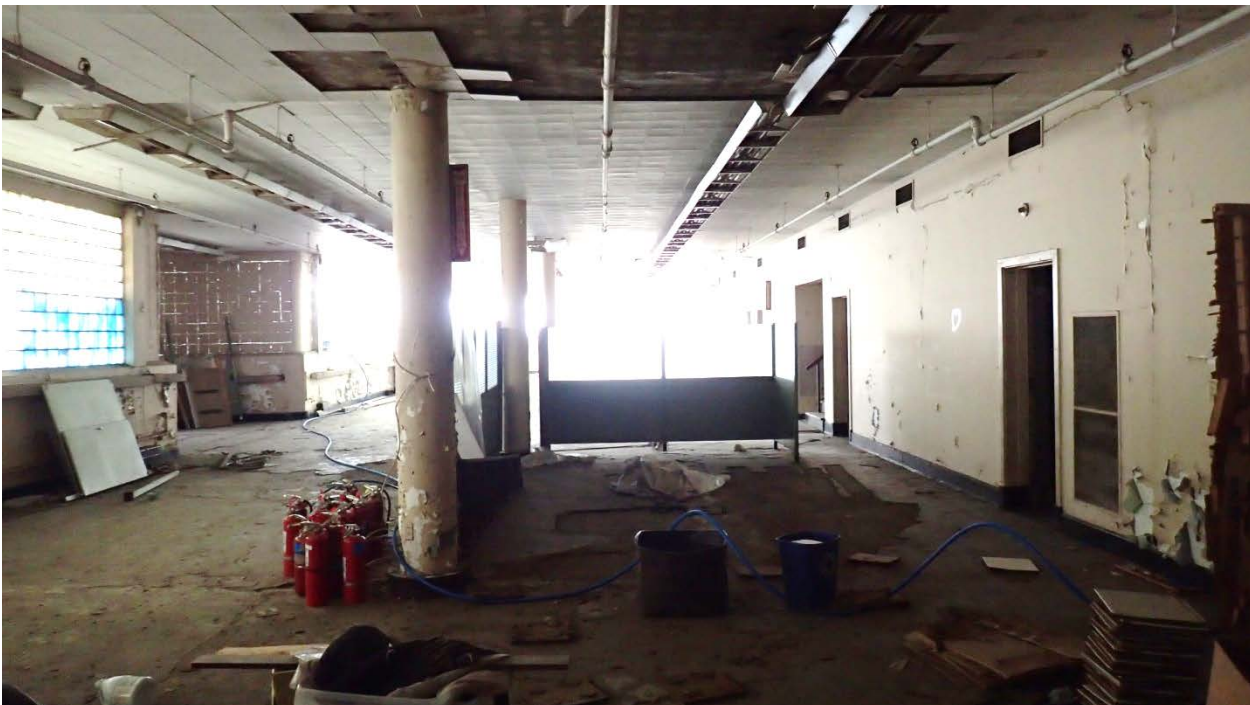
LBC unusable front offices with asbestos containing materials (floor tiles and gypsum board and mastic)
