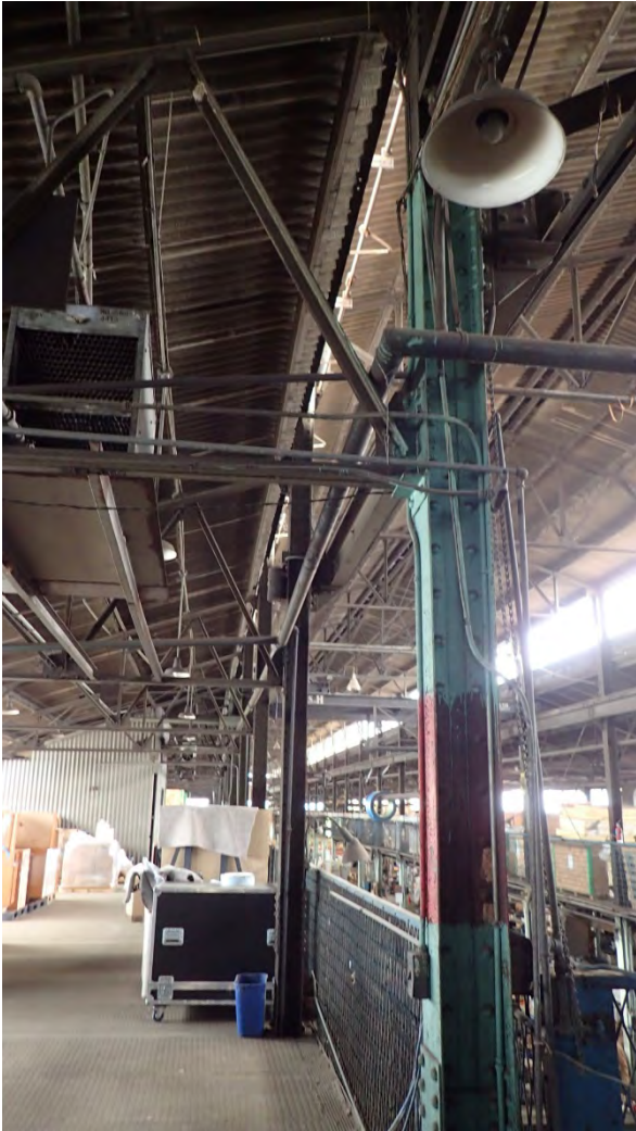
LBC mezzanine level with asbestos containing materials (corrugated Transite) and lead paint pictured
